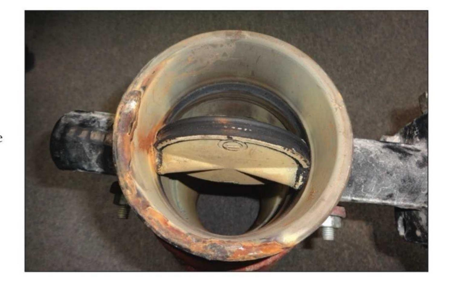
These three pictures show a heavily scaled valve from a luxury hotel in Las Vegas. The same valve just eleven weeks later and another valve from the same hotel three years after Aqua-Rex was installed. The contrast between the "habitat friendly" scaled valve and the "no place to hide" cleaned valve could not be greater.
