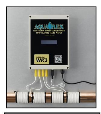
two aerials on the right make up the other pair. Each aerial of each pair must be wrapped in opposite directions from a central point. When facing the pipe, one aerial should start by passing behind the pipe and the other should pass in front of the pipe. Secure each end of the aerial with the zip ties provided.
